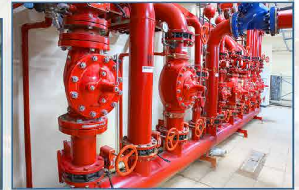
Central Fire Extinguishing,Working Presswe 18,5 Bar
